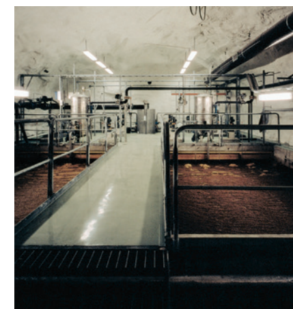
Flofilters under backwash and in operation.
