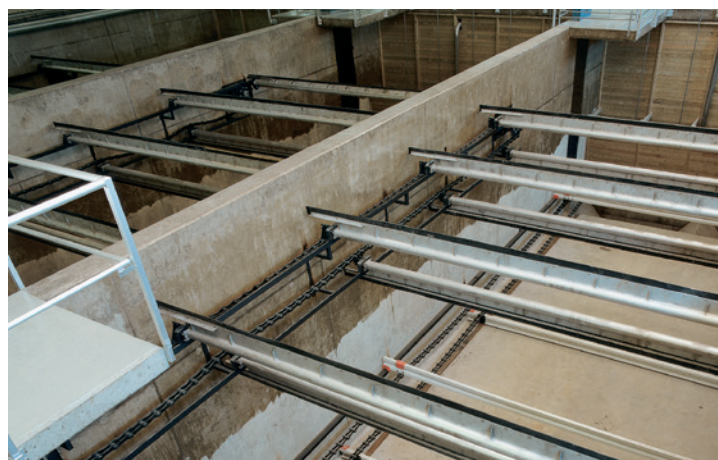
Chain-driven flight scraper for surface sludge removal.
