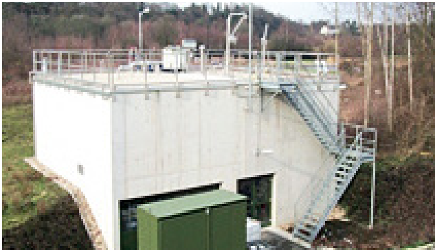
Hattingen wastewater treatment plant, Germany
