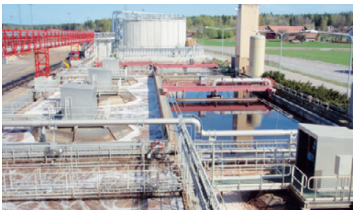
Stora Enso Fors AB Pulp Mill, Sweden
