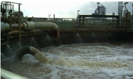
Stenal Pulp Mill, Germany
